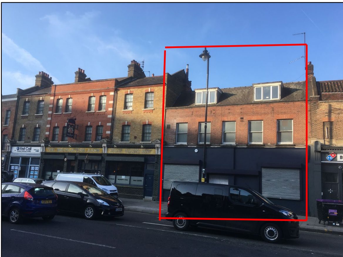
Existing High Road frontage
